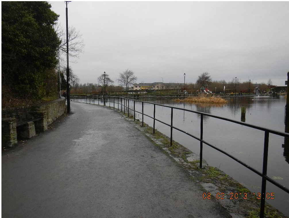
Photo 3.3 Bound surface dressing in Maynooth
