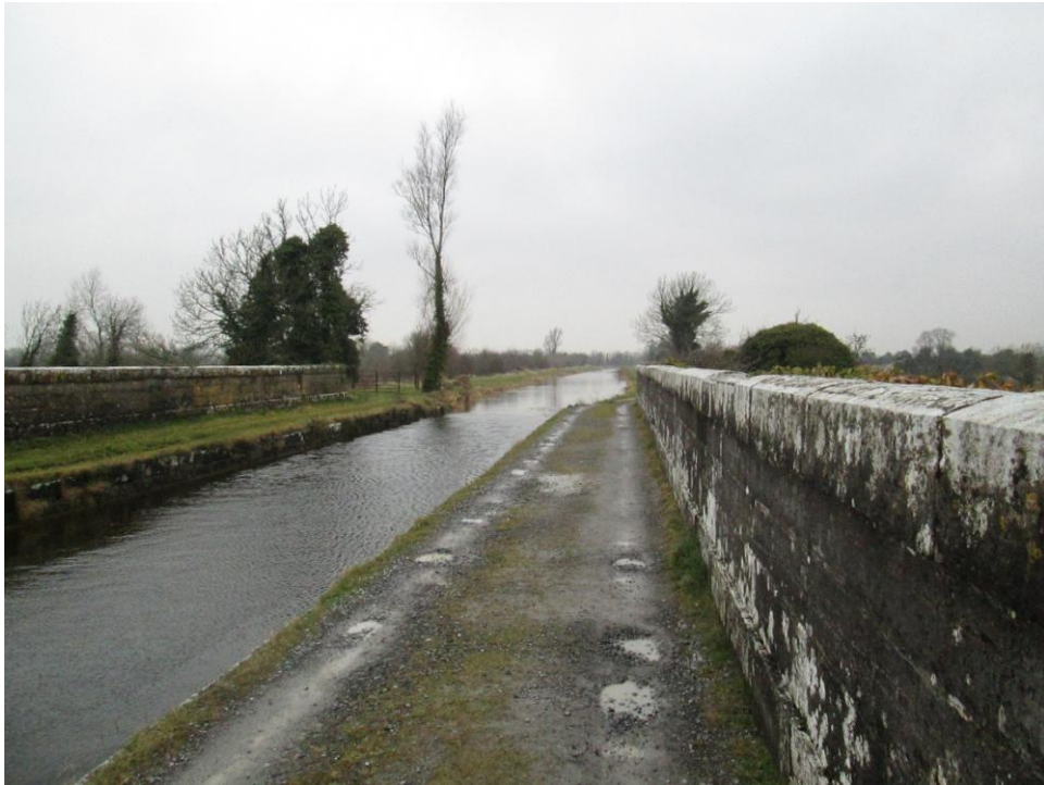
Photograph 5.4 Royal Canal crossing over the River Boyne (Boyne Aqueduct)
