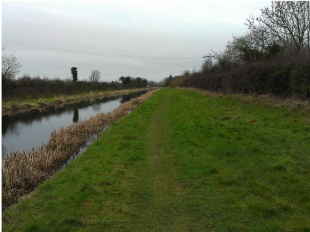
Photo 3.1 Typical managed towpath without vehicular access to be dressed with Quarry Dust
