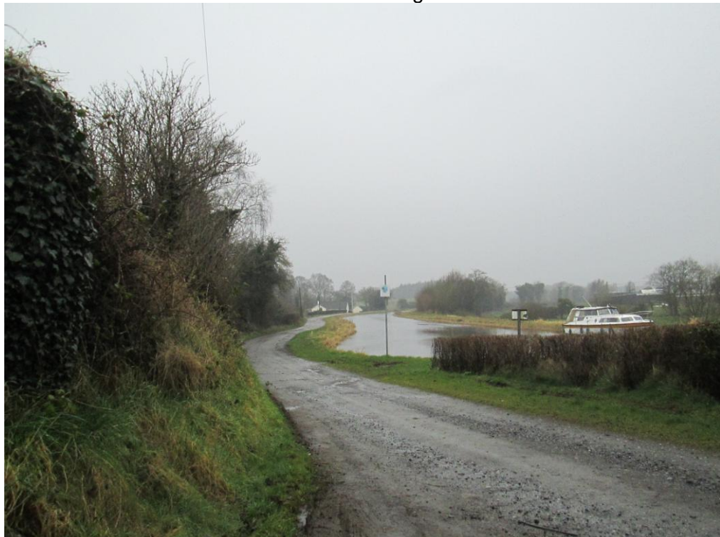
Photograph 3.2 Existing Unbound Surface / Access Road at Ballasport Bridge
